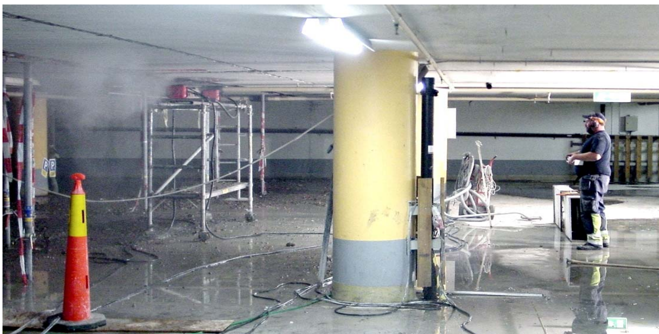
Conjet Jetframe 101 NALTA mounted on standard rolling scaffolding exposing joints in the ceiling of a parking garage. The operator monitors and controls the process at a safe distance from the working area.
