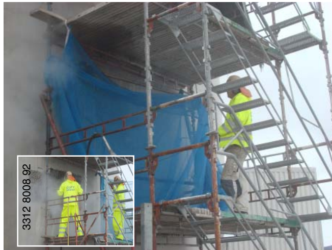
The patent protected Conjet Jetframe 101 NALTA replaces numerous hand lance applications, improving safety and increasing productivity.
